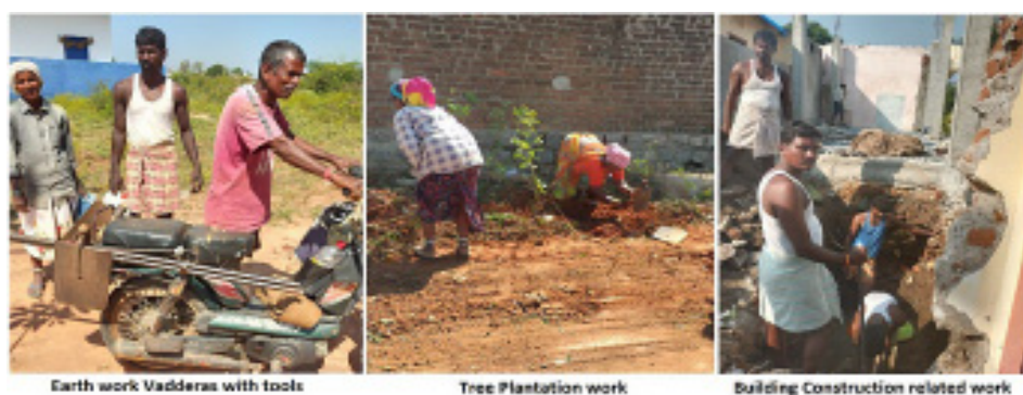
Fig 5.2: Range of activities associated with earthwork
